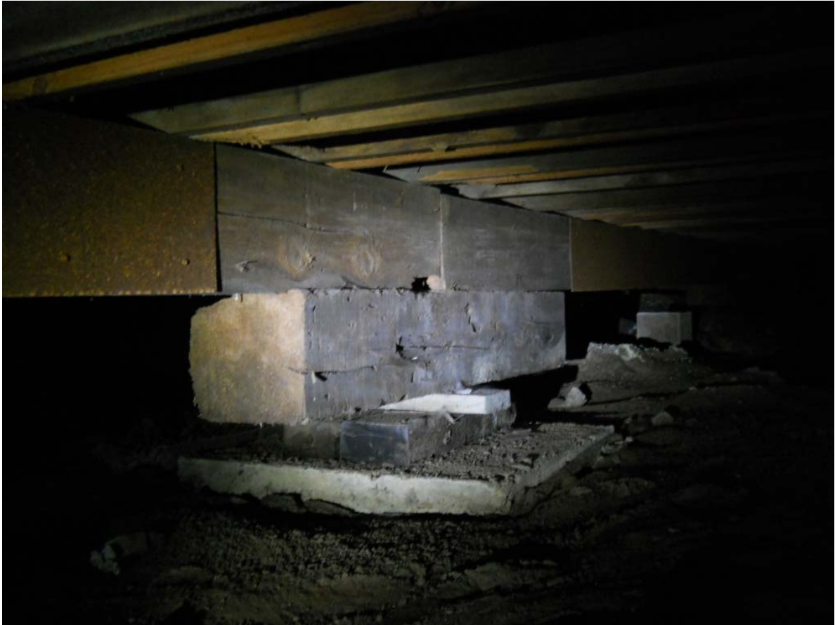
Figure 3: Interior Bearing Beam and Concrete Pier.
