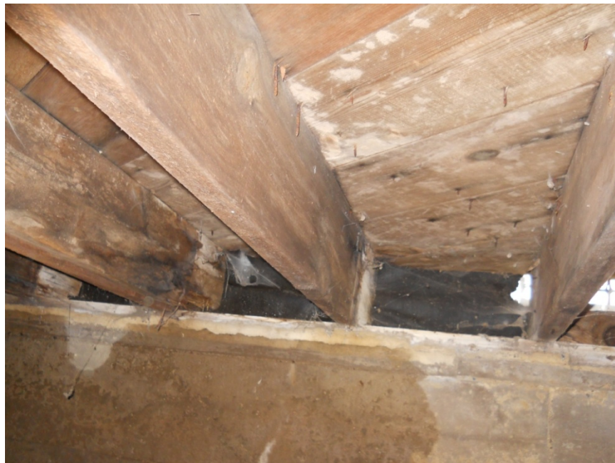
Figure 4: Moisture along inside face of North Wall
