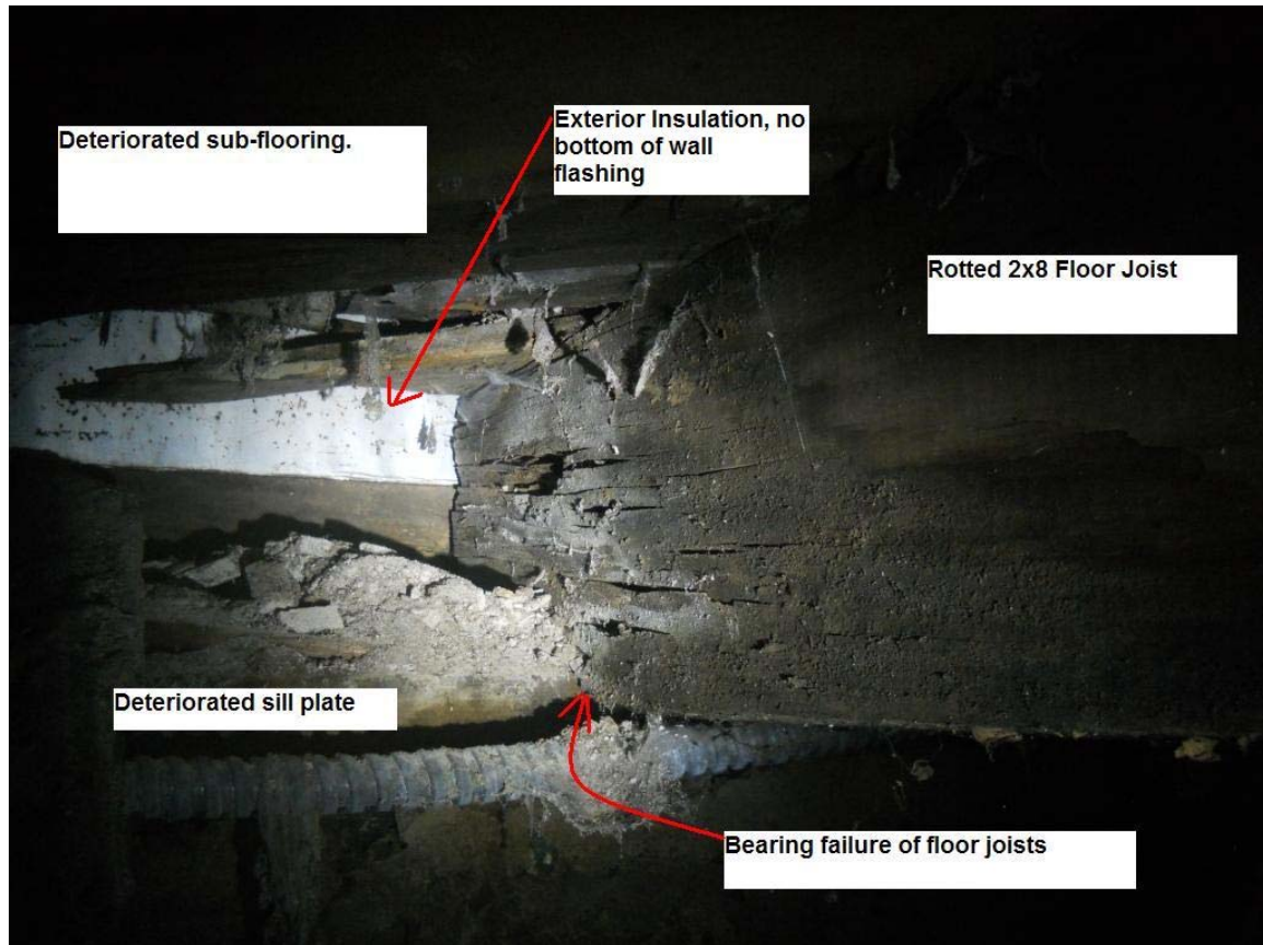
Figure 2: North Foundation Wall with Observations
